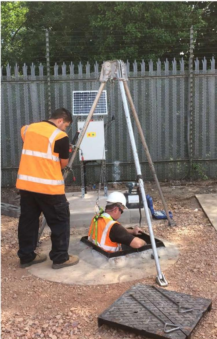
Due to site complexities we installed a solar powered system as running power to the flapstopper would have been problematic.
