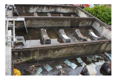
The area the tanks were in was going to be used for redevelopment meaning the entire infrastructure associated with the tanks needed to be removed.
