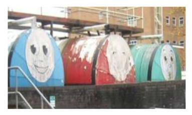
The 45,000 litre tanks had been redundant for several years and contained around 7,000 litres of residual Heavy Fuel Oil inside each tank.
