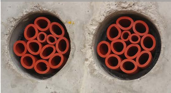
Ducts effectively sealed
