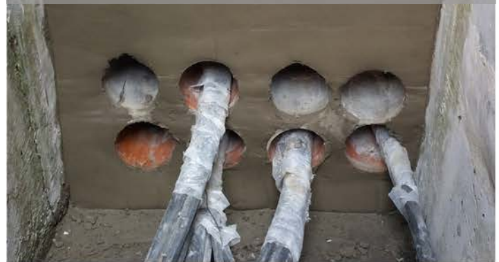
Wall constructed around cables
