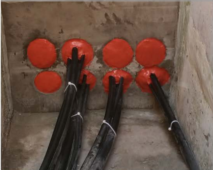
Ducts effectively sealed
