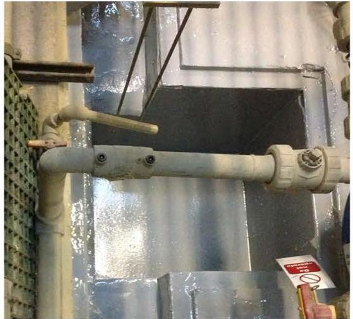
We presented the client with an economical proposal of repairing the damaged areas and relining any areas which were likely to come into direct contact with acids. This meant only relining half of the bund and drastically reducing the timeframe to allow completion within the shutdown period and consequently reducing project costs (whilst still leaving the bund fully compliant).
